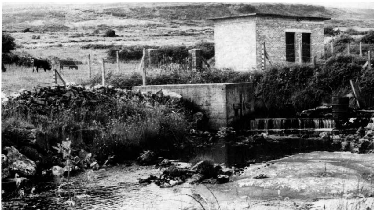
Figure 10. Photograph of the karst spring at Killeany together with the pumping station which withdraws much of the outflow.
