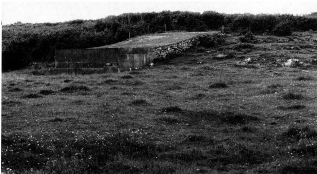
Figure 9. Photograph of an artificial micro-catchment on the Burren designed to collect and store water for use by cattle.
